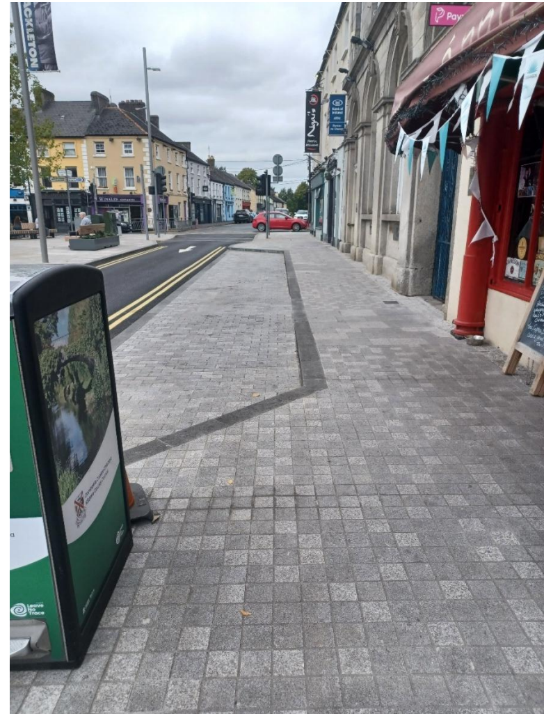
Footpath Improvement After (KCC Inspection July 2025)
